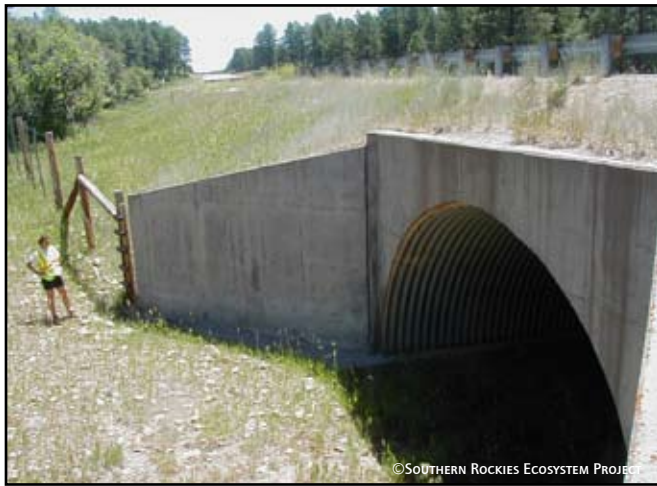
MULTI-PLATE ARCH CONSTRUCTED IN 1973 ON US HIGHWAY 160 NEAR MANCOS, COLORADO.
