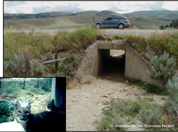
BOX CULVERT ON HWY 13 SOUTH OF CRAIG, COLORADO (ABOVE). BOBCAT USING A BOX CULVERT IN RIVERSIDE, CA UNDER CA 71 (LEFT).
