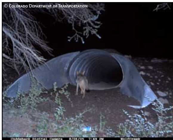
COYOTE APPROACHING AN ELLIPTICAL CULVERT ON WOLF CREEK PASS, US HIGHWAY 160, COLORADO.
